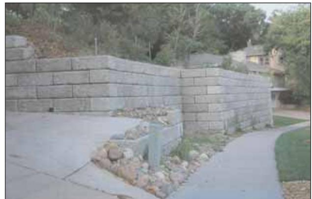
The completed retaining wall eliminated the 1:1 slope 15 ft (4.6 m) from the face of the wall.
